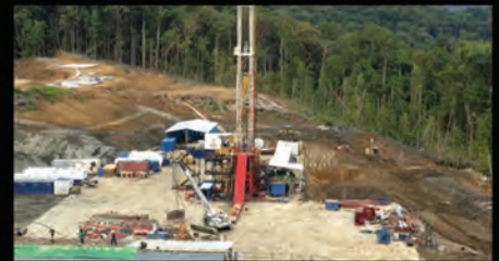
REMOTE SITE CONSTRUCTION
