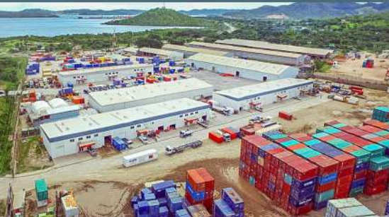
Baruni Industrial Centre
