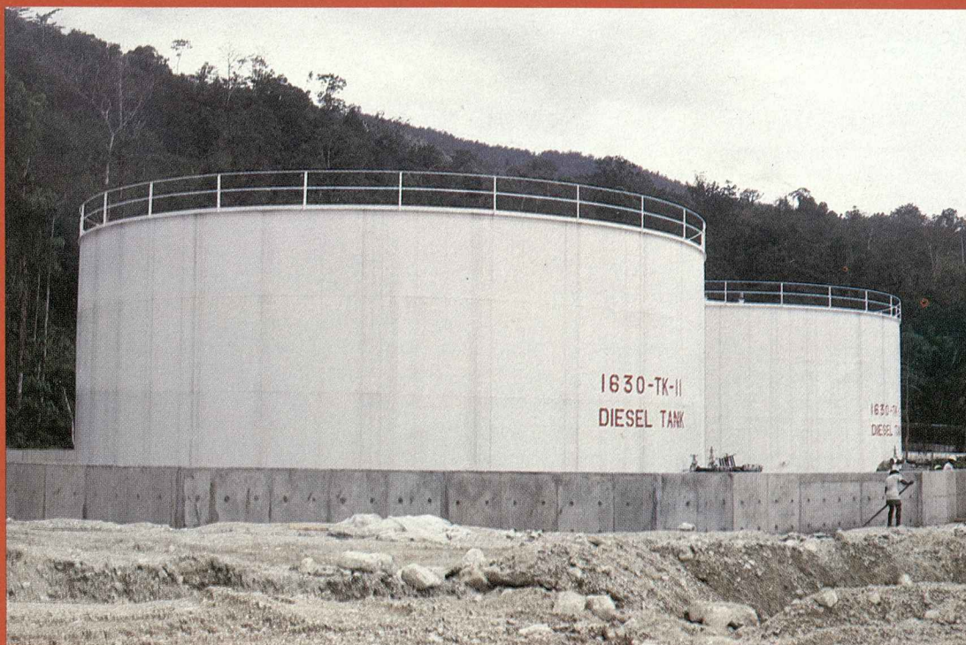
Two tanks - part of a large installation of bulk storage at Kiunga and Tabubil, Papua New Guinea for OTML. Construction by NGI Steel. Tanks contain water and diesel fuel. Protective treatment of internal and external surfaces included Zincilate 120 - inorganic zinc silicate primer, top coated with Armourcote 418 and Amercoat 383HS - high solid epoxys.
