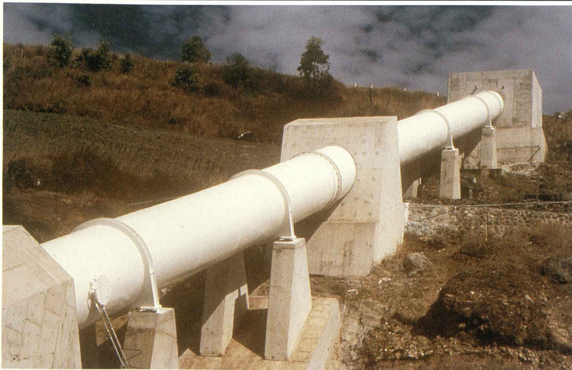
A section of Rouna 4 Penstock, near Port Moresby. 2.2 metres diameter, 300 metres long. Internal surfaces treated with 400 micron film thickness of Tarsel, Standard tar epoxy. External surfaces 75 micron film thickness of Dimetcoat 5, inorganic zinc silicate and 75 micron of Unilite 400, poly vinyl chloride. Application by: Hornibrook Constructions Pty Ltd.
