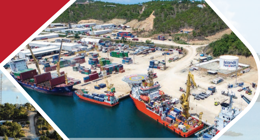
Port and Supply Base
