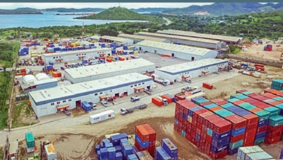
Baruni Industrial Centre
