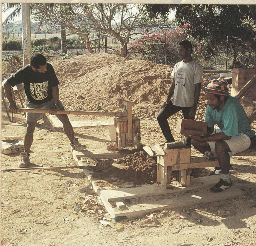
Top Mud bricks and mortar quickly become a wall. left Bubble level indicates accuracy of the brickworks. below Two Cinva rams can produce hundreds of bricks a day.
