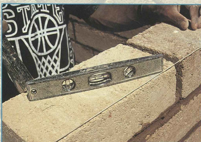
Top Mud bricks and mortar quickly become a wall. left Bubble level indicates accuracy of the brickworks. below Two Cinva rams can produce hundreds of bricks a day.
