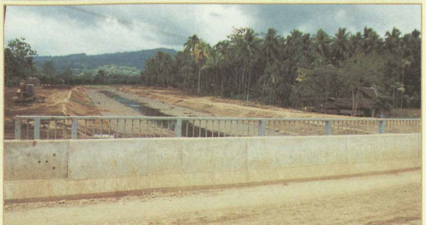
For efficiency, this bridge was built, then the river diverted from its usual bed to flow under the bridge.
