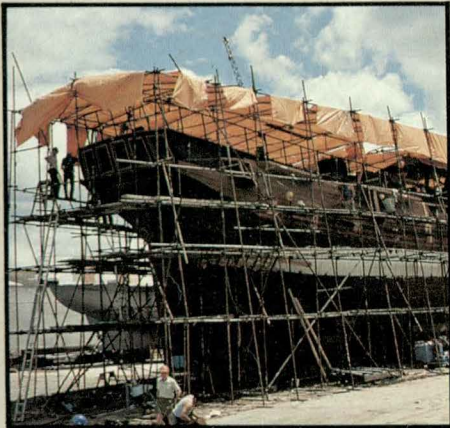
An all steel hull . . .
