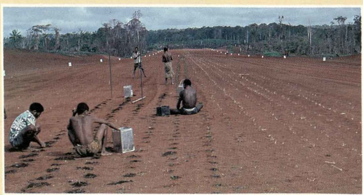
Many hands . . . and still it's hard going carving out a Highlands airstrip. Sometimes a tractor, assembled on site, is available to help, but usually it's all done by picks, shovels, axes and wheelbarrows — and much sweat of the brow
