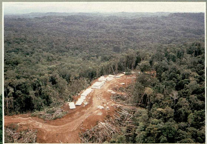
Fuel and plant equipment for the project is barged over 1200 km to Kiunga from Port Moresby; inset anti-clockwise from above: road construction from Tabubil to Mt Fubilan; road gangs sleep on the job in temporary camps; the road was cut through 135 km of virgin bush; traditionally the way to cross the raging streams in the mine area
