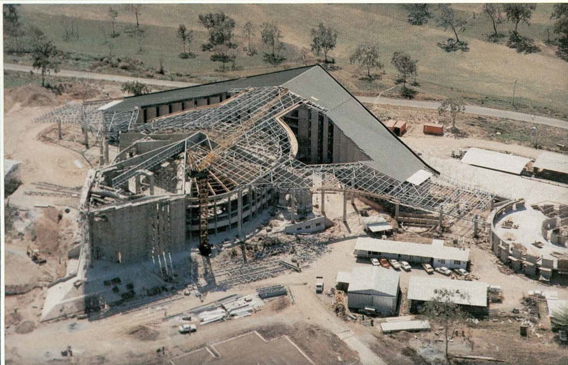
Parliament House - Port Moresby Roof Steelwork fabricated and erected by Hornibrook Constructions Pty Ltd. Protection Treatment: Abrasive Blast clean to Australian Standard 1627.4 Class 2.5 followed by Dimetcote 5 Inorganic Zinc Silicate to 75 micron dry film thickness.
