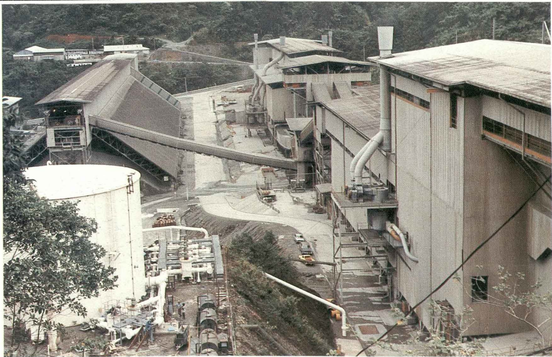
A section of the Bougainville Copper Limited's Panguna installation. Dimet high performance coating systems protect structural steelwork and plant. Application by Bougainville Protective Coverings Pty. Ltd. (PNG).
