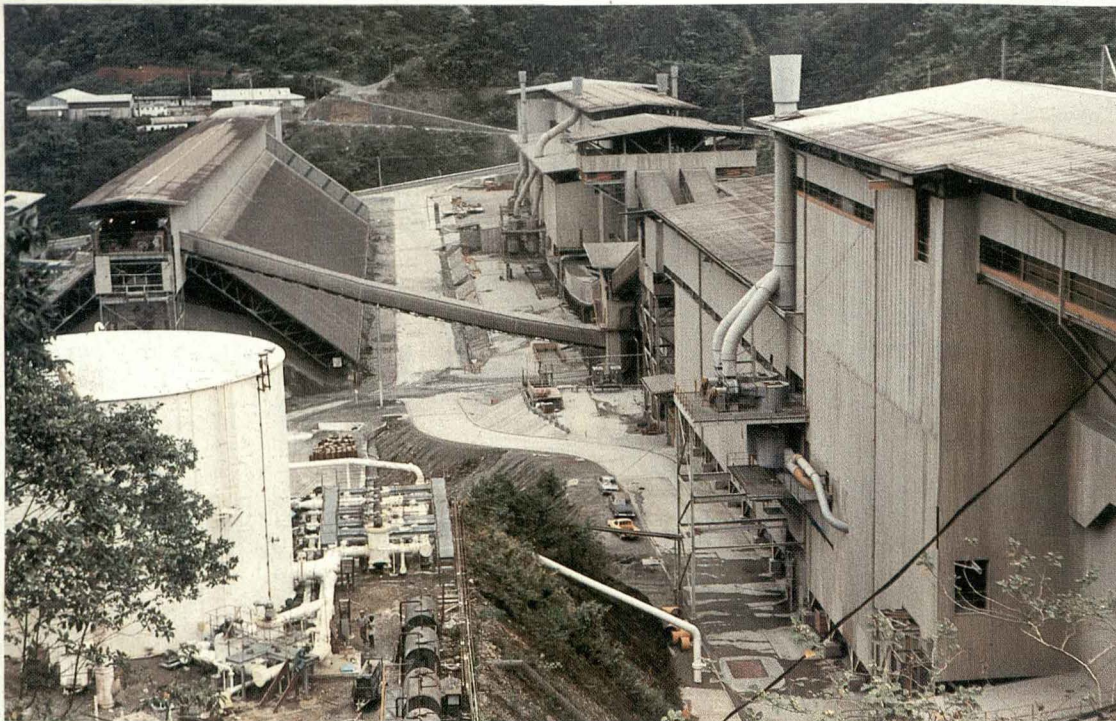
A section of the Bougainville Copper Limited's Panguna installation. Dimet high performance coating systems protect structural steelwork and plant. Application by Bougainville Protective Coverings Pty. Ltd. (PNG).
