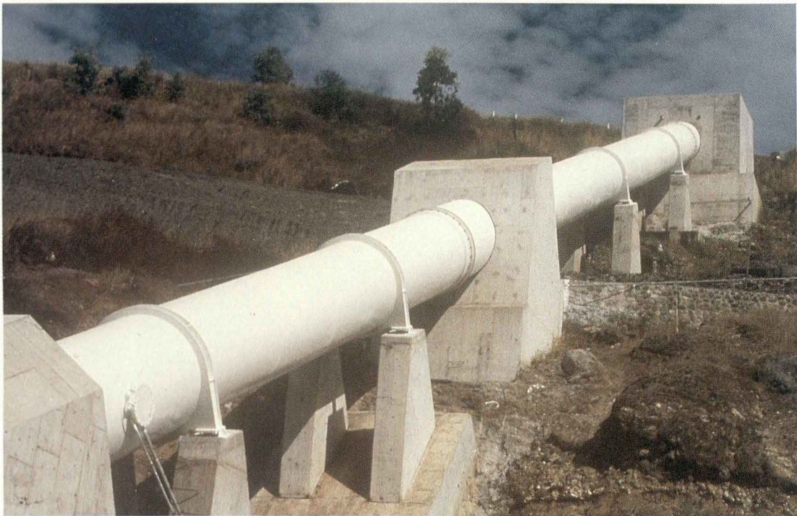
A section of Rouna 4 Penstock, near Port Moresby. 2.2 metres diameter, 300 metres long. Internal surfaces treated with 400 micron film thickness of Tarsel, Standard tar epoxy. External surfaces 75 micron film thickness of Dimetcote 5, inorganic zinc silicate and 75 micron of Unilite 400, poly vinyl chloride. Application by: Hornibrook Constructions Pty Ltd.
