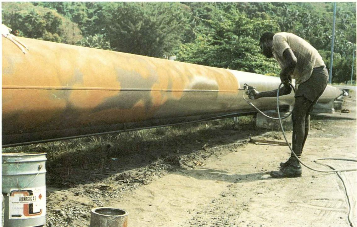
Dimet corrosion control in action. Fuel Oil Supply Line at Loloho Bougainville. Treated with Alumastic an aluminised fibre reinforced protective mastic coating. Application by airless spray 250 micron dry film thickness.
