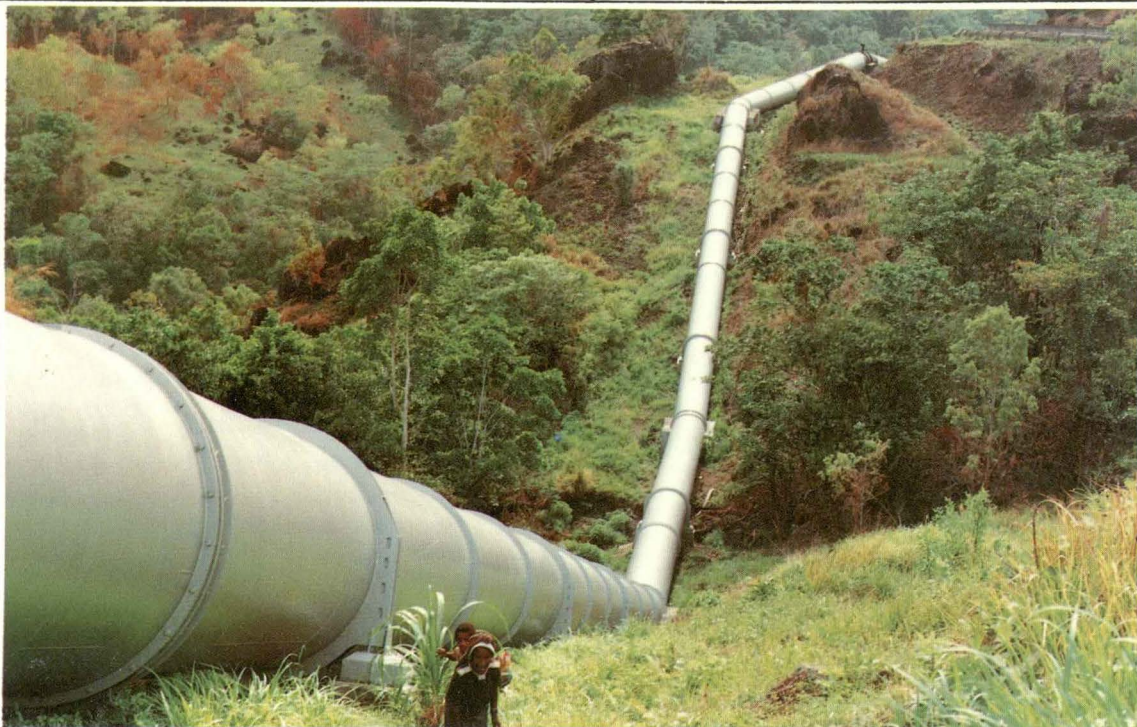
A section of the Rouna 3 water pipeline near Port Moresby. External surfaces treated with Amerlock 400 high build epoxy mastic applied in two coats to 250 micron dry film thickness.
