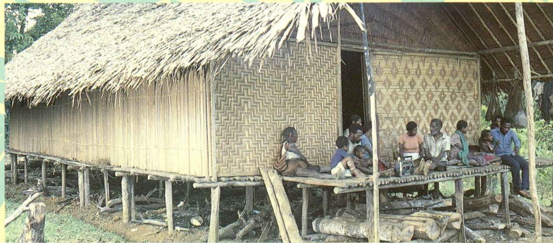
Inset above Paring sago pith. top Sago making trough. bottom House with sago thatch roof and plaited sago frond walls.
