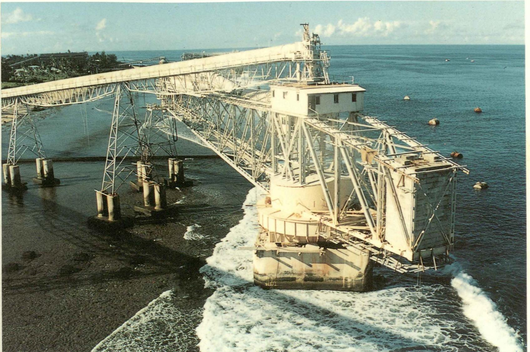
"Cantilever loading facilities at Nauru; All steelwork treated with Dimet High Build Epoxy Coatings to 300 Micron Dry Film Thickness. Application with airless spray equipment over abrasive blast cleaned surface preparation."
