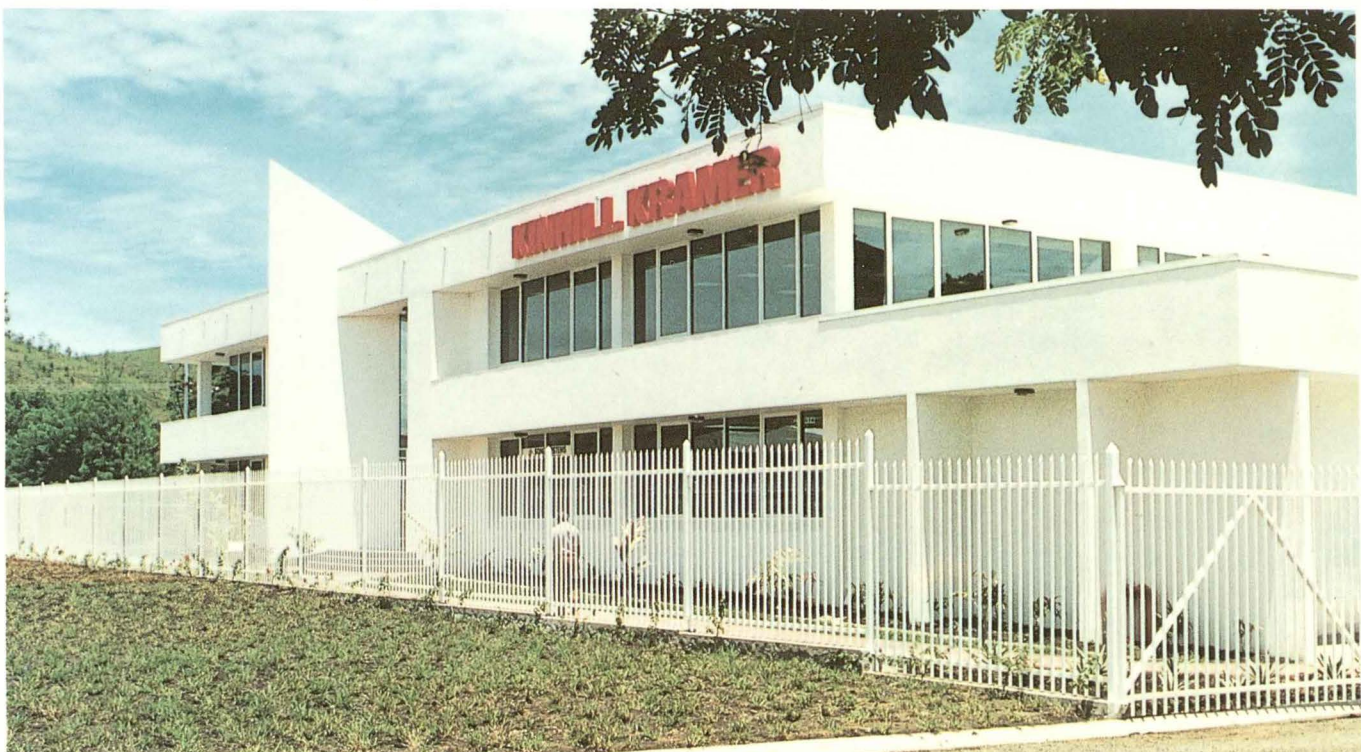
Kinhill Kramer offices Port Moresby – designed by Peddle Thorp Architects, received the "Papua New Guinea Institute of Architects Award of Merit for Good Design."
