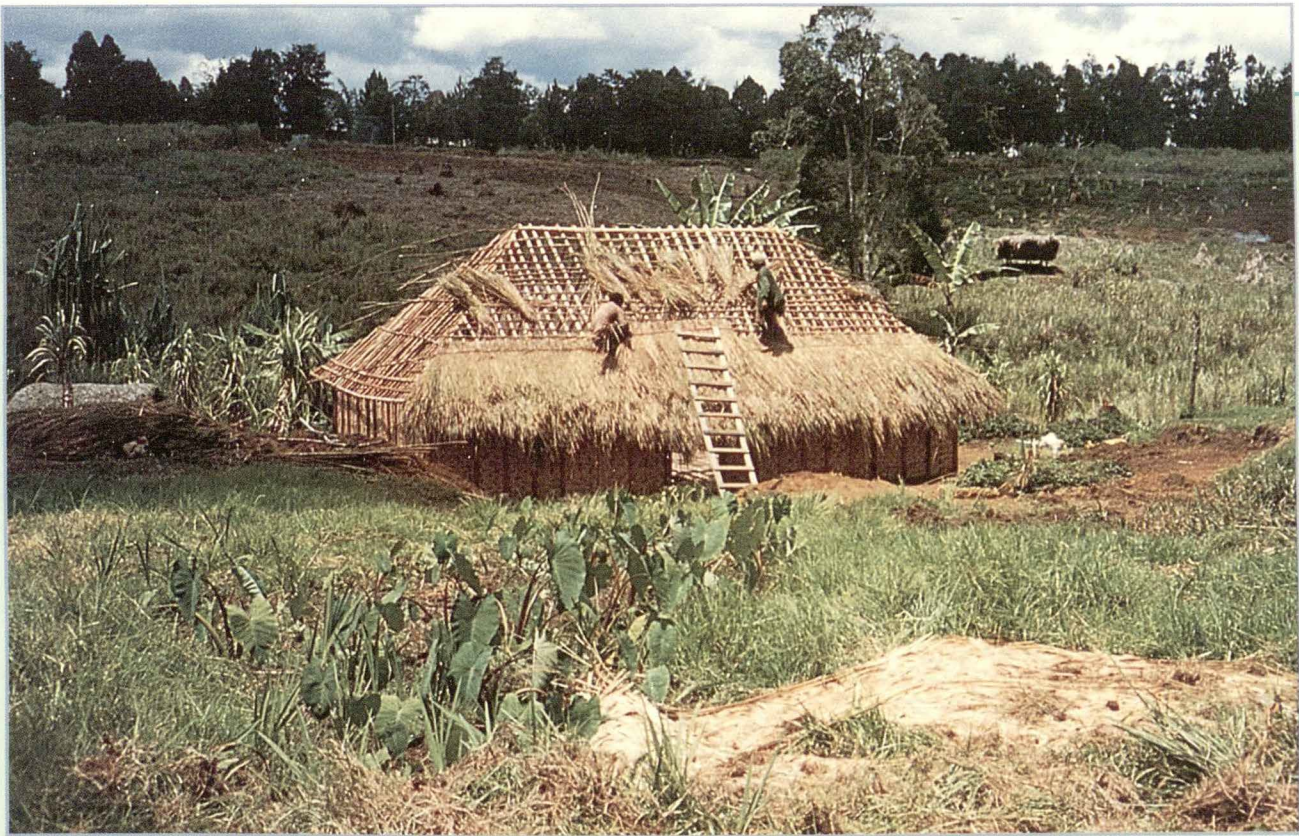
Above Thatching a roof with kunai grass. right Framework takes shape.
