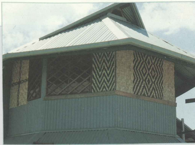
Left Award-winning design in East New Britain. centre left Bamboo ceiling in modern house. centre right Informal structures which inspire the new breed of architecture. bottom Informal structure showing modern influences.
