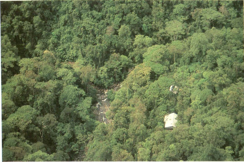
The Wara Sera Research Station is nestled within virtually undisturbed lower montane and hill rainforest. The station consists of a 12 x 16m structure raised on 2.5m stilts which can house six researchers comfortably, with a smaller 'writer's cabin' situated further up the mountain side which can accommodate two more.
