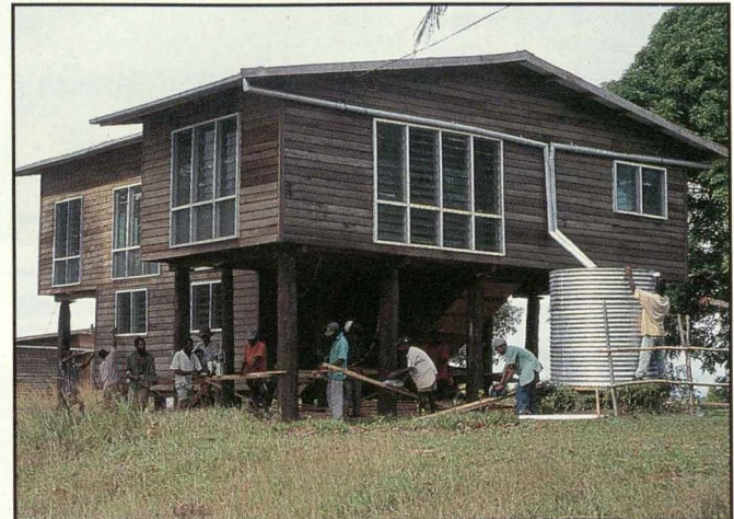
Below: New teacher's house being built by Biyama Trading Company carpenters.
