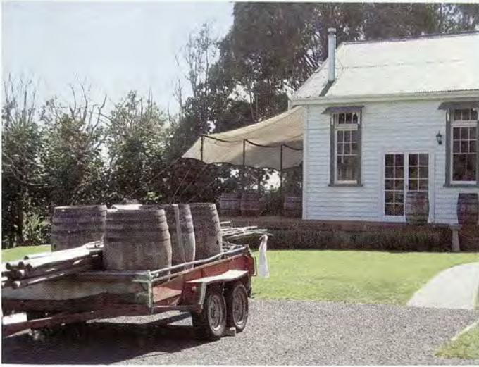
An 1880's schoolhouse...reconverted to a function centre.
