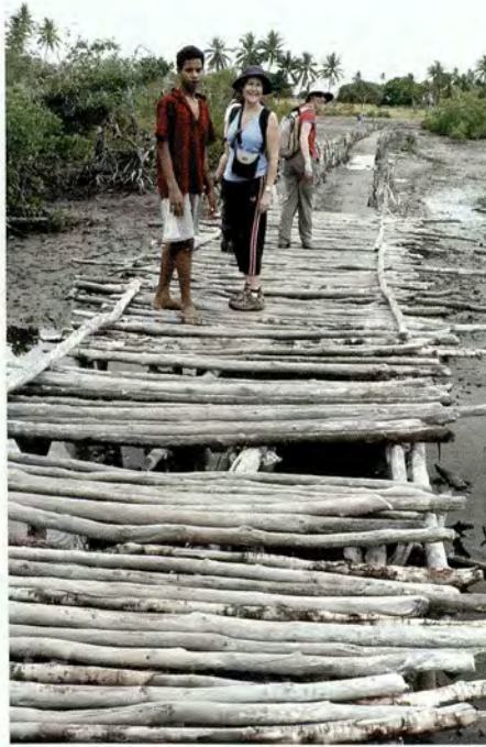
Swamp bridge crossing.
