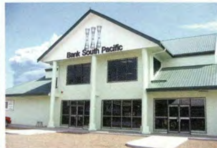
BSP Bank Kokopo Project
