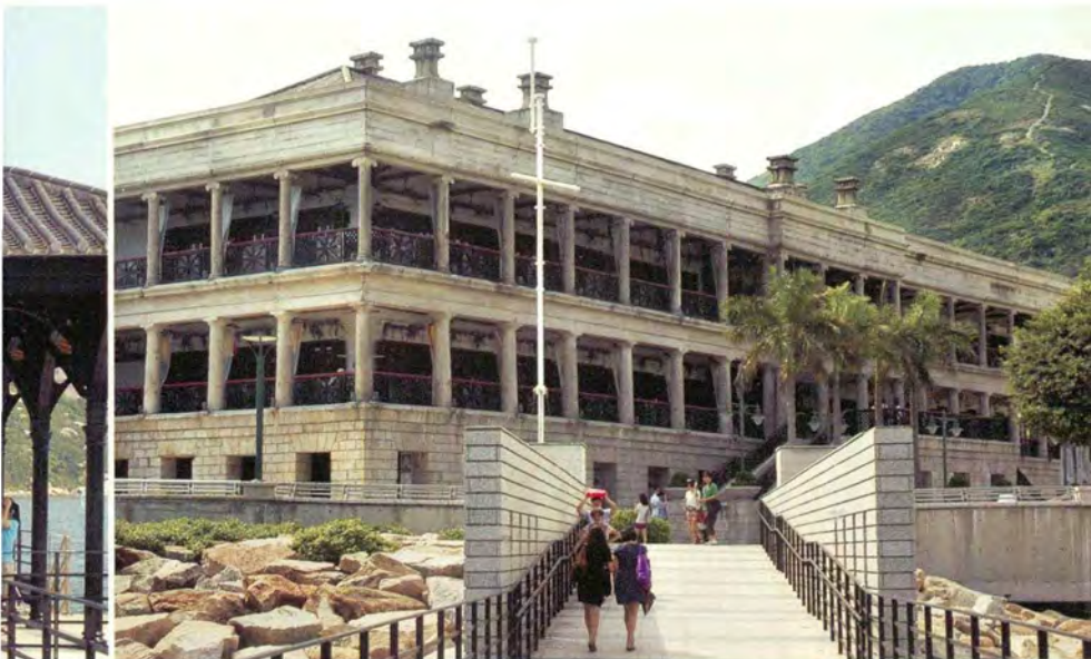
Murray House...one of the oldest European military buildings on Hong Kong.
