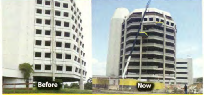
High Rise Construction
