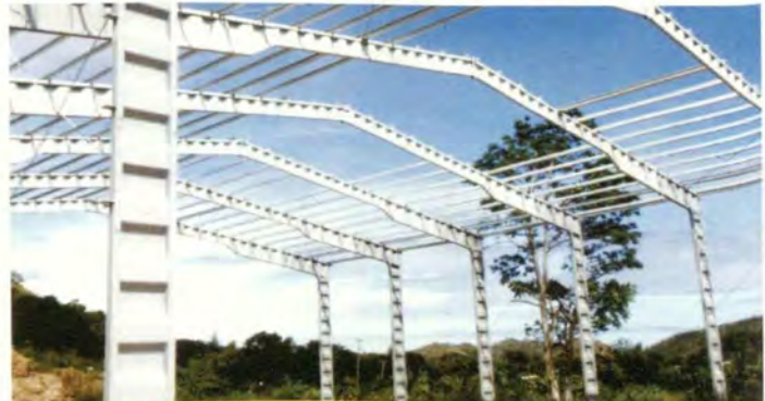
Steel Fabrication (ILB)
