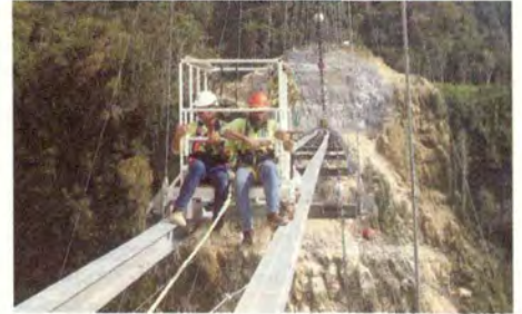
Maintenance techs crossing the bridge trolley.
