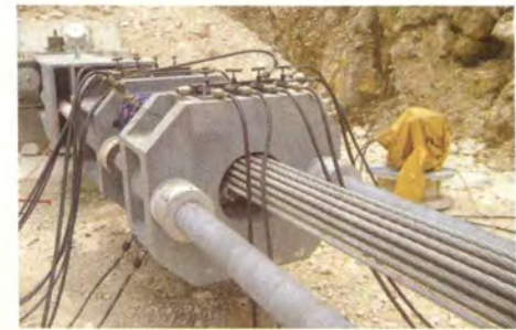
Rock anchor detail.
