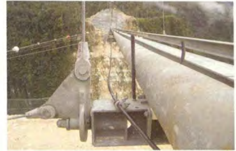
Looking across pipelines on the bridge.
