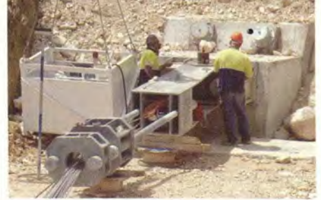
Rock anchor under construction.
