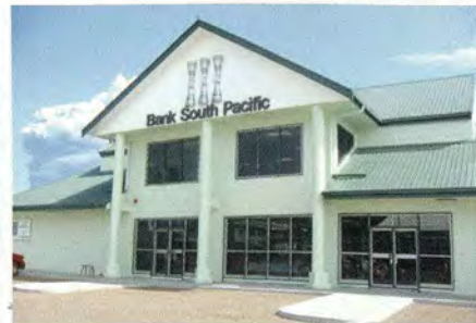
BSP Bank Kokopo Project
