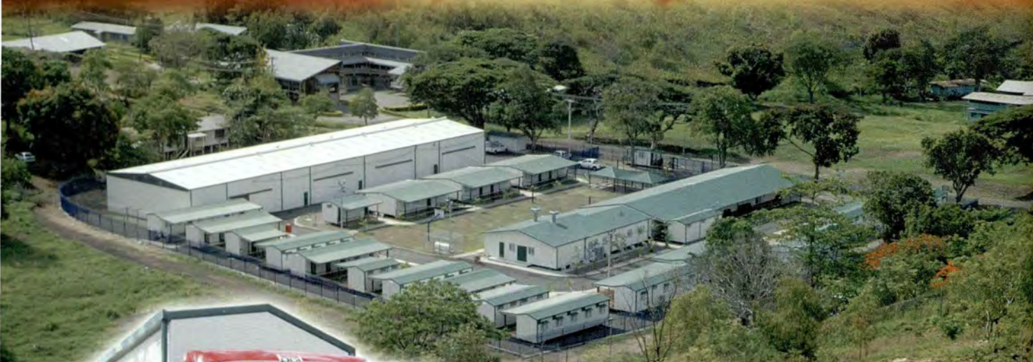
APTC Campus Port Moresby-Designed and Built by API Buildings.
