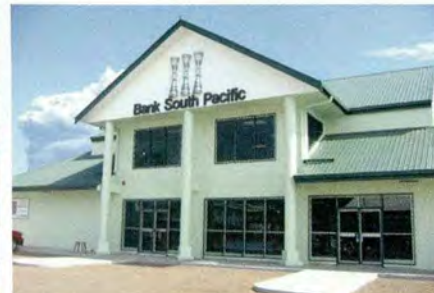
BSP Bank Kokopo Project
