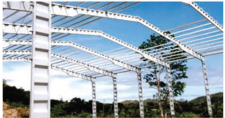
Steel Fabrication (ILB)
