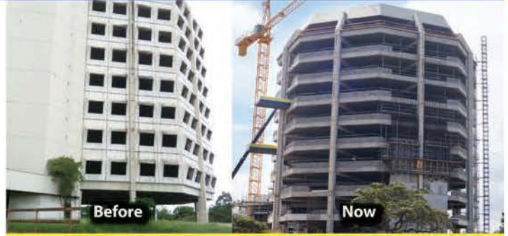
High Rise Construction
