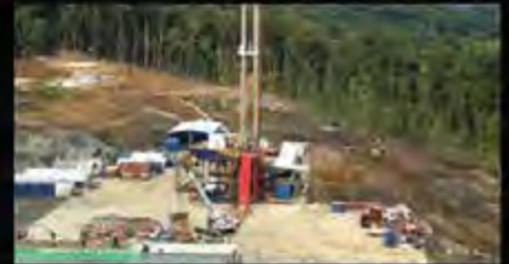
REMOTE SITE CONSTRUCTION
