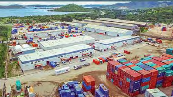
Baruni Industrial Centre
