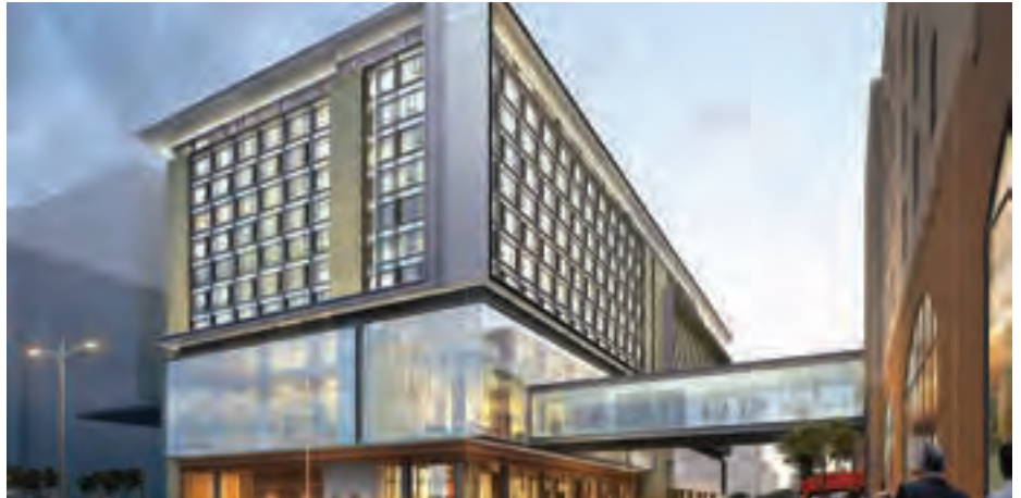
Hilton Manila ... connected by skybridge to the airport (above); luxurious interiors and the lagoon pool (opposite page).
