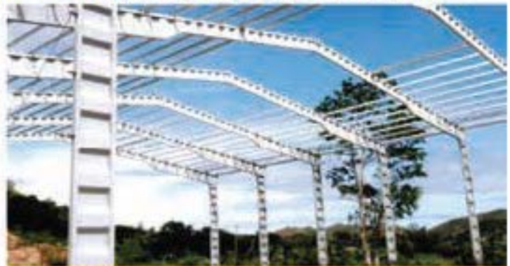
Steel Fabrication (ILB)
