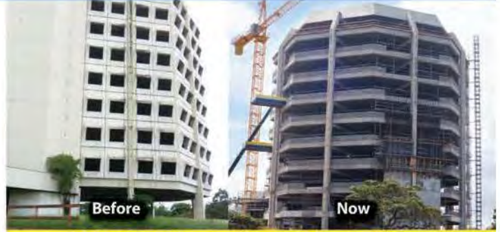
High Rise Construction
