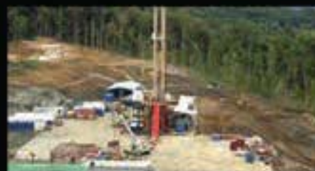
REMOTE SITE CONSTRUCTION
