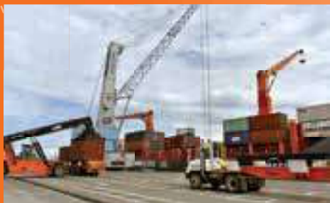
Being the largest container handling facility in PNG, the Port of Lae has become a major port of call—mainly through SPICTL's expansion of port facilities, and complementary development programs that include hiring of locals from the port's host communities.
