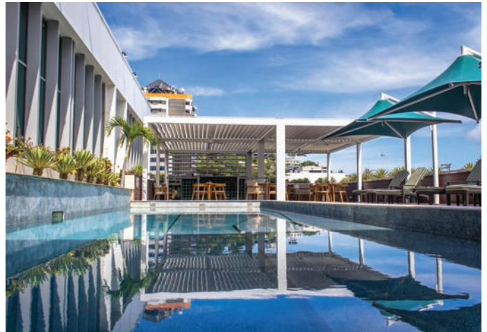
The renovated pool deck at the Grand Papua Hotel, where the Coral Sea Hotels group is spending up to PGK80 million on a major rejuvenation.
