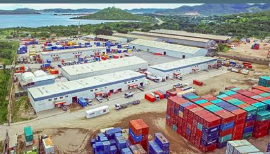
Baruni Industrial Centre
