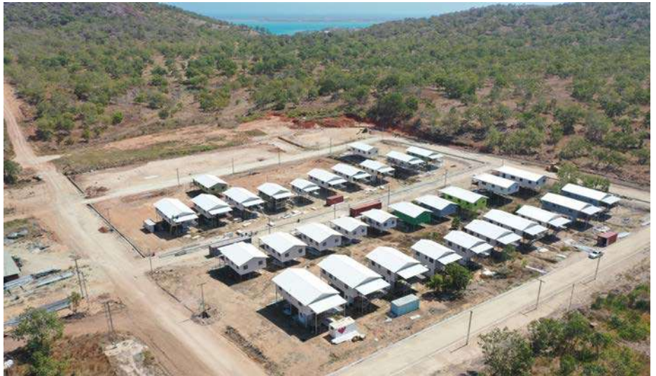
Taking shape, the first houses at Tuhava town.
