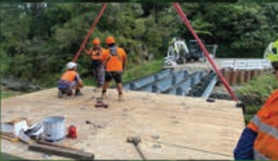
NiuDeck installation, New Zealand
