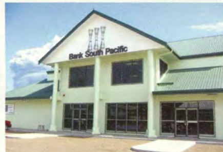
BSP Bank Kokopo Project
